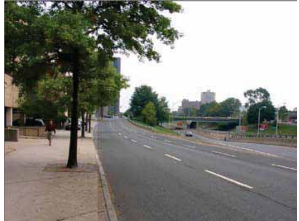
View of the Existing Route 34 Corridor.
